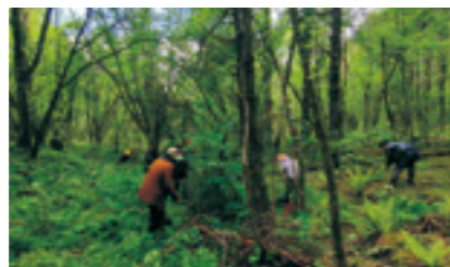
Forest and irrigation clearing at Xiaoxiangling project site
